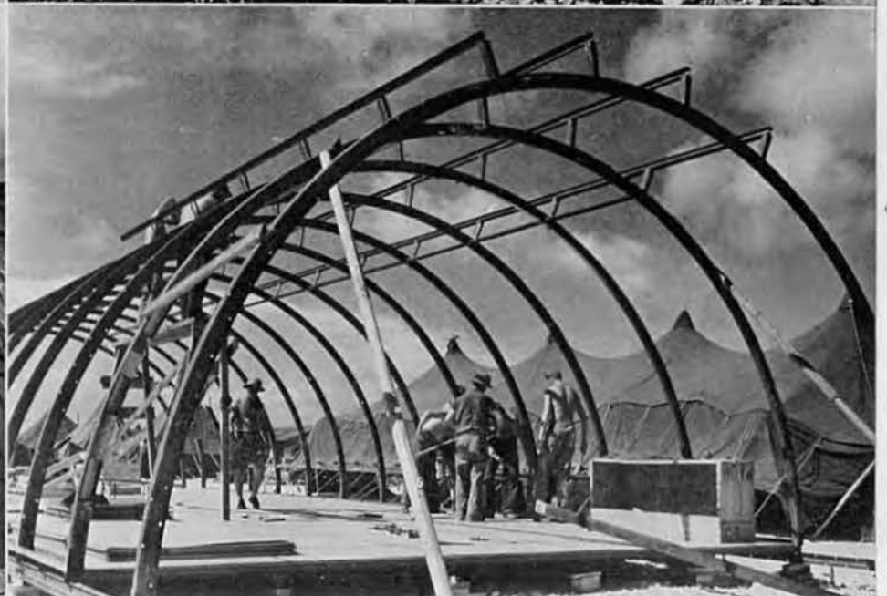
Top—Torpedo Hut Near Completion. Bottom—Quonset Hut Framework.
