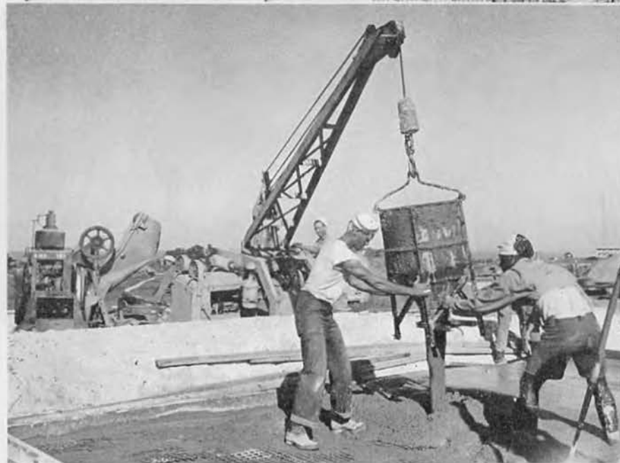
Top—Fuel Tank Aboard 6x18 Pontoon Barge. Bottom—Concreting Foundation for H-20 Tanks.
