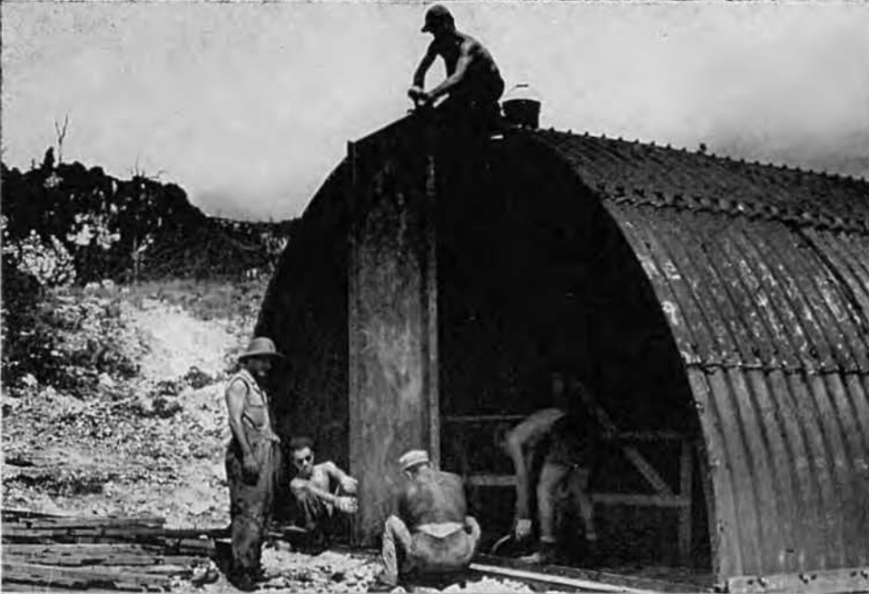
Top—Laying Concrete Deck. Bottom—Erecting the Bulkhead.
