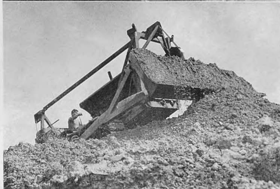
Top—Drag Line Excavation. Bottom—Loading Barge Members.
