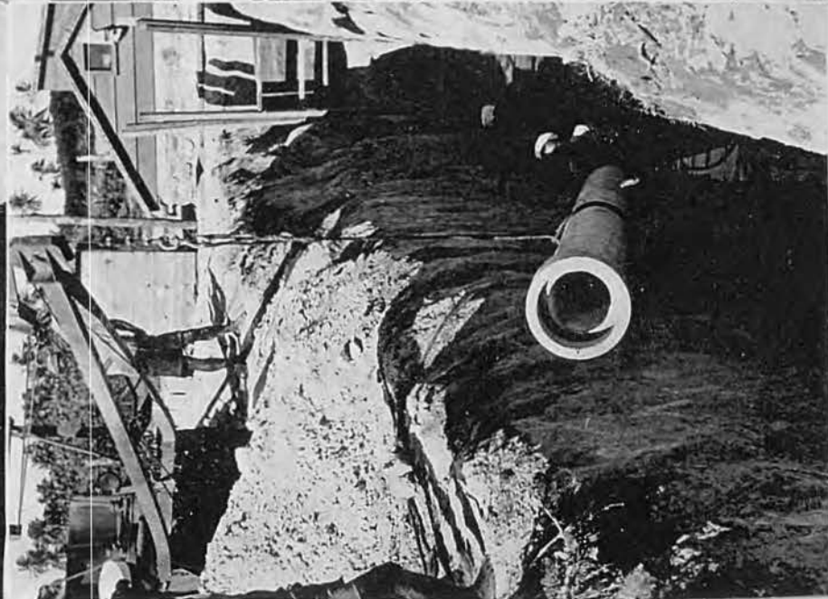
Top—Placing Wells Retaining Walls. Bottom—Laying Perforated Pipe to Collect and Carry Water to Well.
