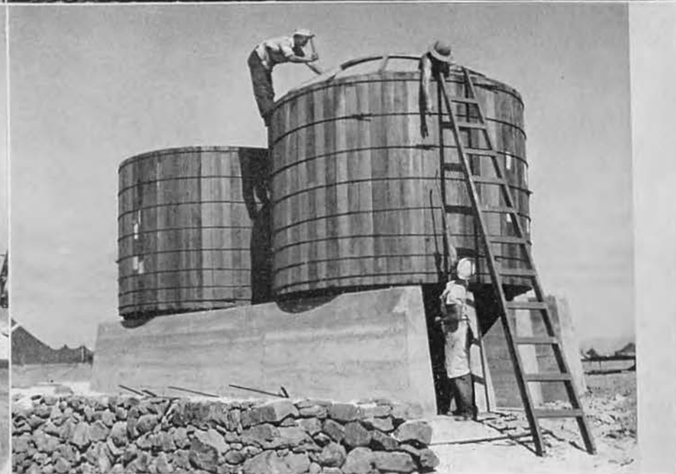
Top—Erecting Tank Aboard Barge. Bottom—Assembling Wood Tanks for Water Storage.
