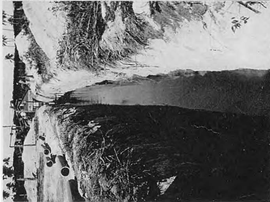
Top—Excavating Coral Pit Well. Bottom—Trench to Facilitate Drainage to Well.
