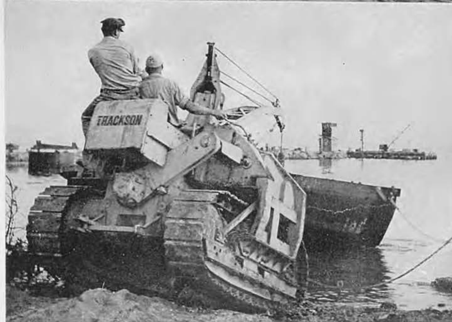
Top—Initial Push to Launch. Bottom—Launched Section Is Righted.
